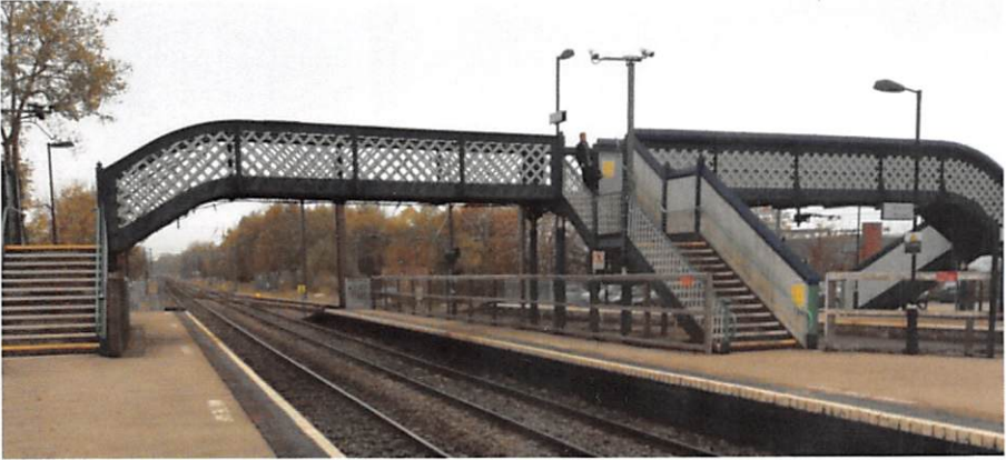
The existing footbridge at Barnt Green station which will be replaced
